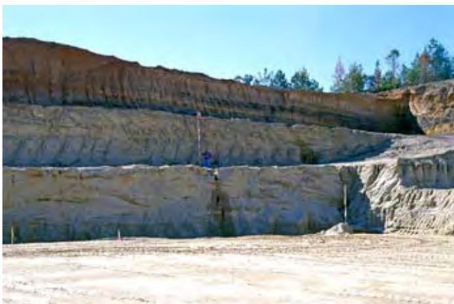
Figure 11. Ken Davis holding survey rod on a channel sand in the lower Hatchetigbee Formation at the construction side of a Super Wal-Mart in Meridian, Mississippi. Here the channel sand is about 30 feet thick and comprises the excavation floor and two benches in the high wall. Picture (slide 341-14) taken on October 13, 2000.
