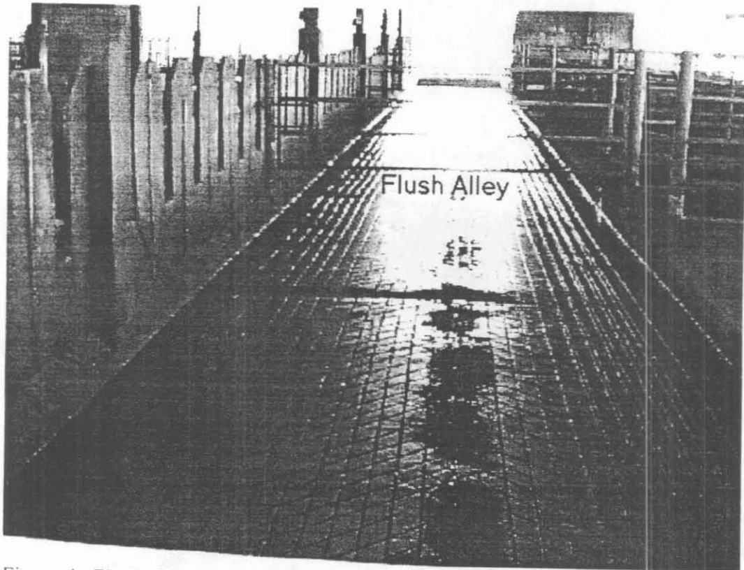
Figure 4. Flush alley in free-stall barn.
