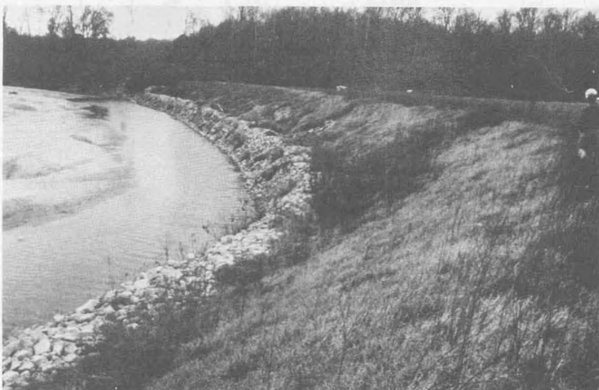
Figure 21. Longitudinal Stone Dike with Upper Bank Seeding
