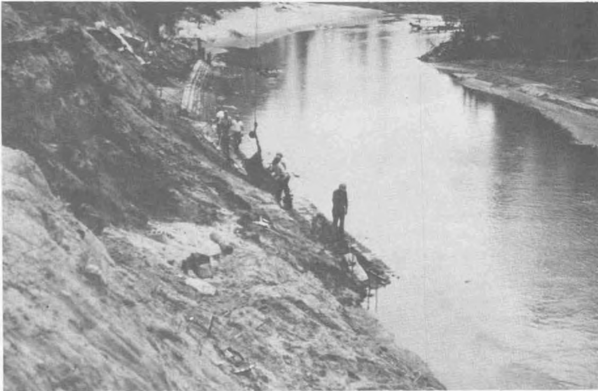
Figure 18. Placing Soil Cement Sack Revetment
