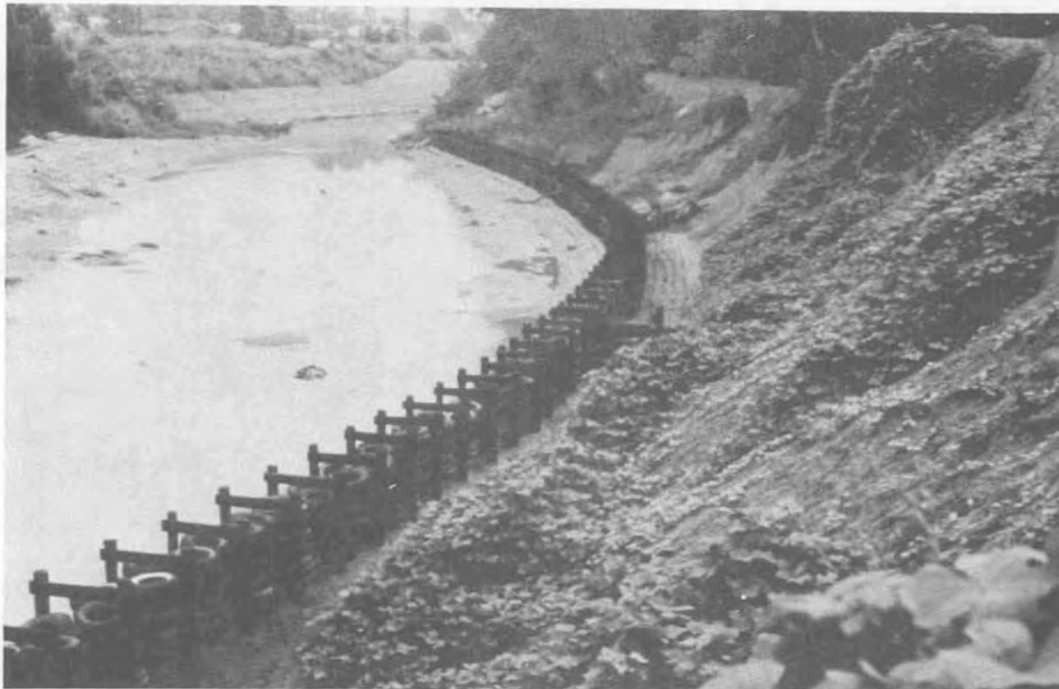
Figure 12. Longitudinal Toe Protection Using Used Tires
