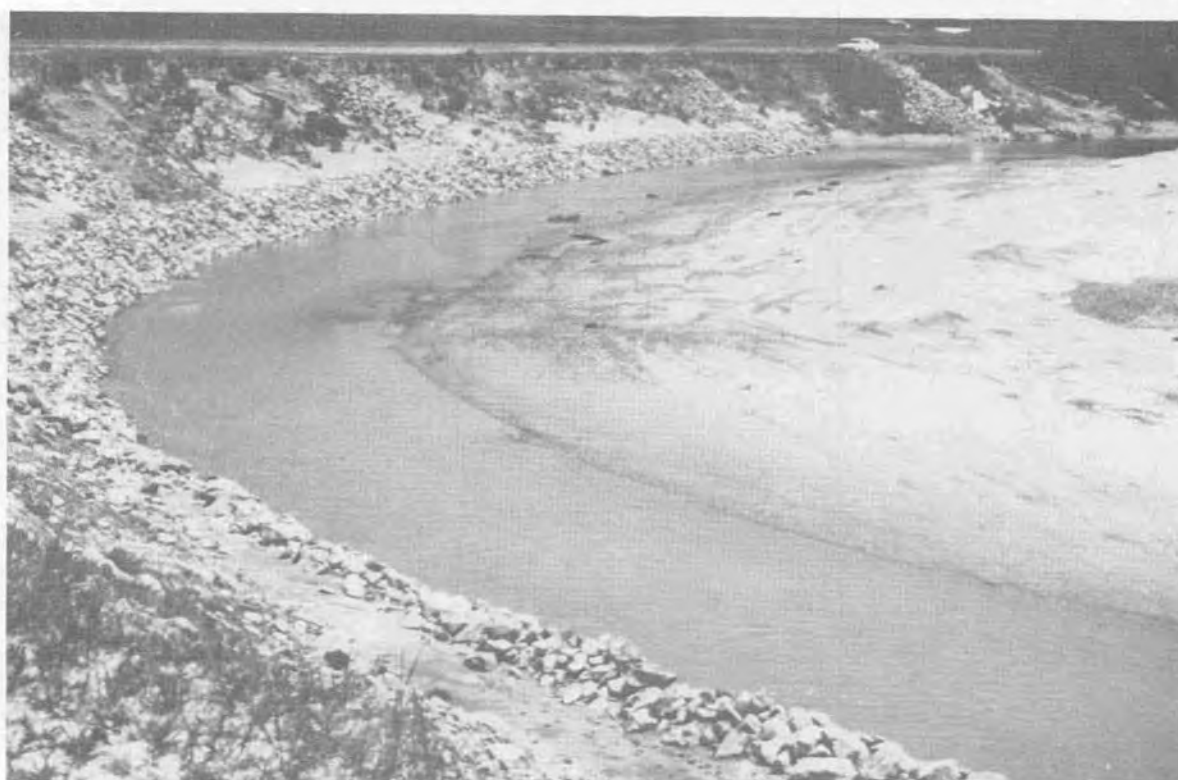
Figure 11. Longitudinal Stone Dike with Tie Back
