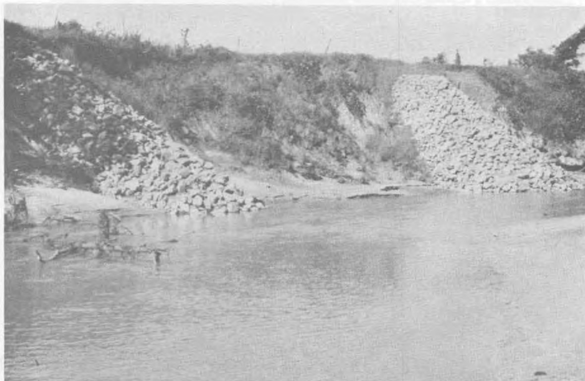
Figure 8. Transverse Stone Dike
