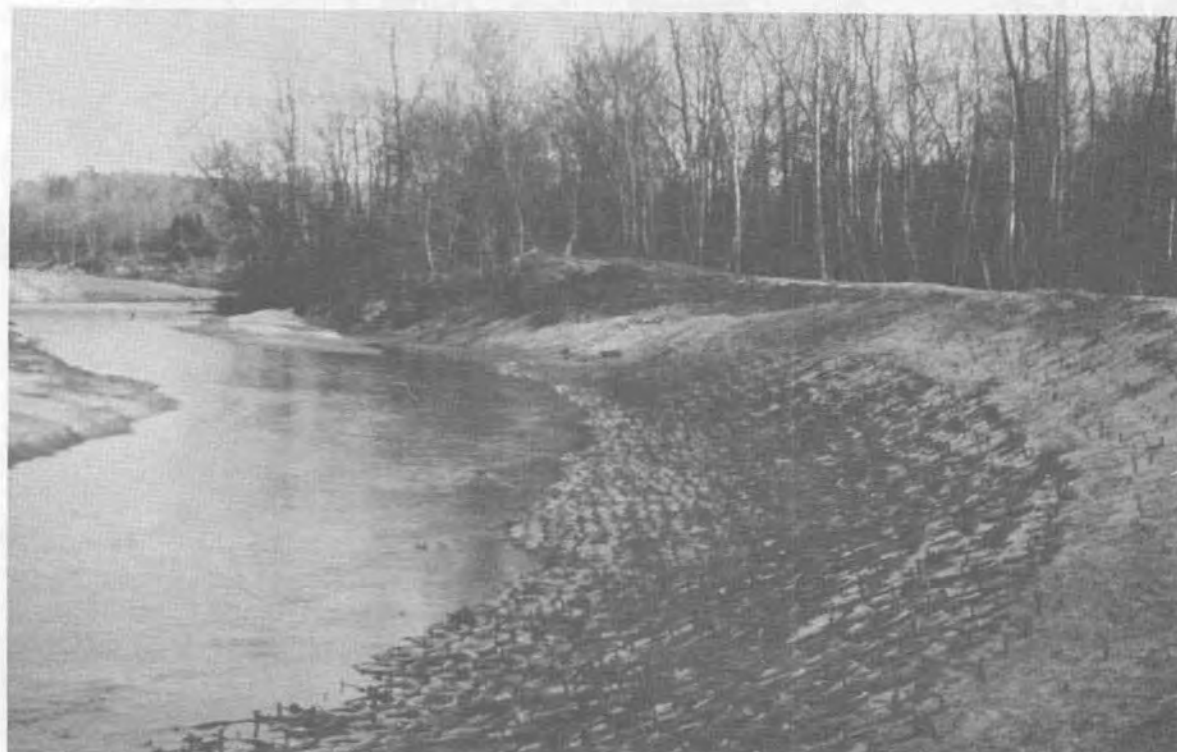
Figure 7. Used Tire Revetment with Willow Stob
