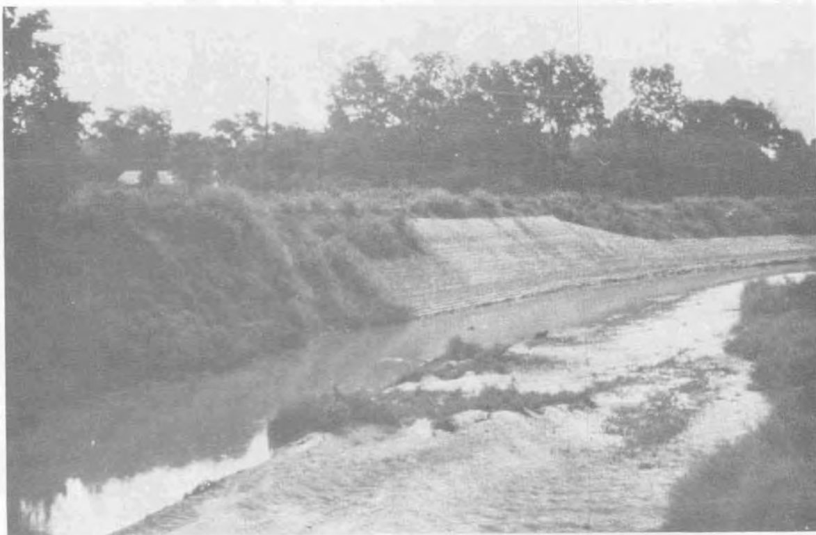
Figure 19. Soil Cement Sack Revetment in Place
