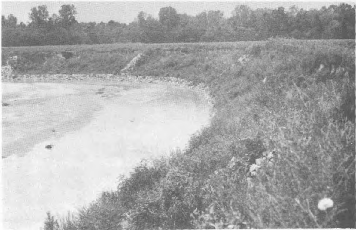
Figure 17. 2 Years After Longitudinal Stone Dike with Tie Back
