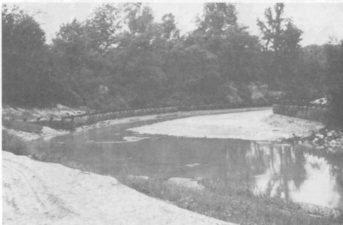
Figure 13. Longitudinal Toe Protection Using Hay
