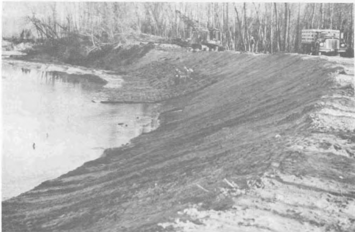
Figure 14. Placing Used Tire Revetment with Willow Stobs
