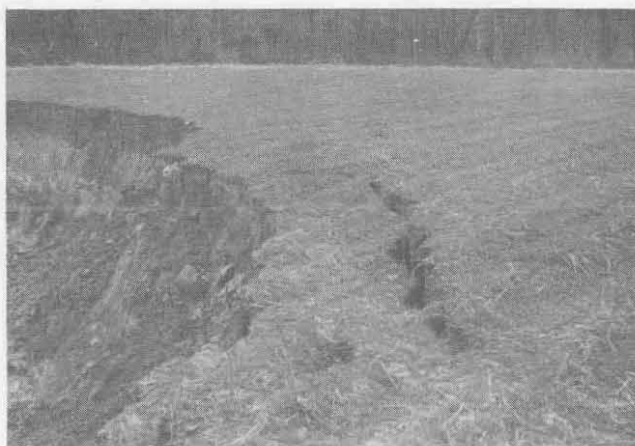
Fig. 18. Tension Crack in Top Bank
