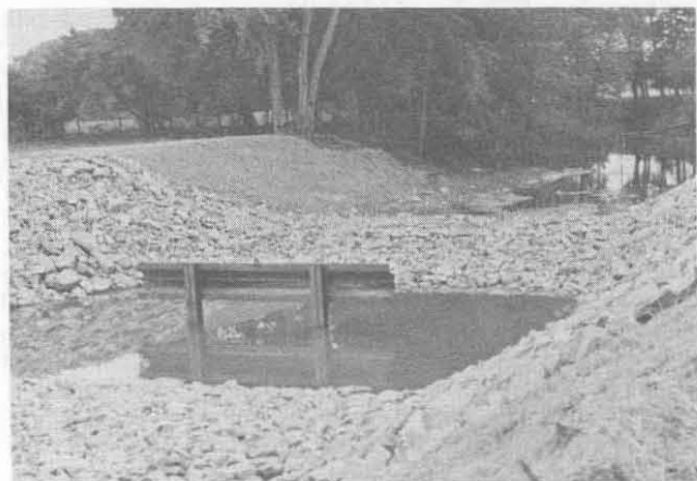
Fig. 20. Grade Control Structure - Perry Creek
