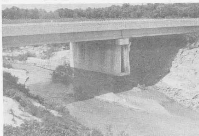
Fig. 1. Degradation at Bridge Site - 1 Year After Completion
