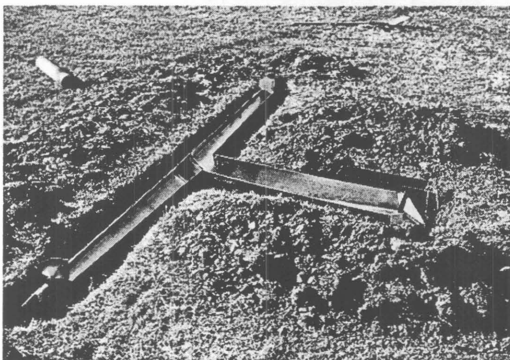
Figure 4. Installation of collector, approach, HS-flume, and electronic stilling well.
