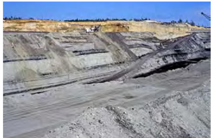
Figure 8. A channel sand in the lower Tuscaloosa Formation at the Red Hills Lignite Mine underlies the J seam and, at right, cuts out the I and H2 seams. The G and F seams can be seen bending beneath the channel sand where they intersect the ramp ascending from the quarry floor. Picture (slide 393-38) taken on November 10, 2004.
