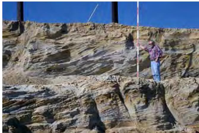
Figure 12. Ken Davis holding survey rod on a bench cut into the cross-bedded channel sands of the lower Hatchetigbee Formation at the construction site of the Super Wal-Mart (power pole site) in Meridian (view is to the west). Picture (slide 341-5) taken on October 13, 2000.
